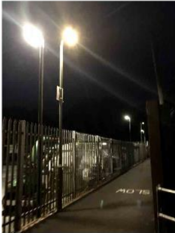
Looking along the public footpath linking Barfield Close with Domum Road, the lamp posts are estimated to be 8m high
