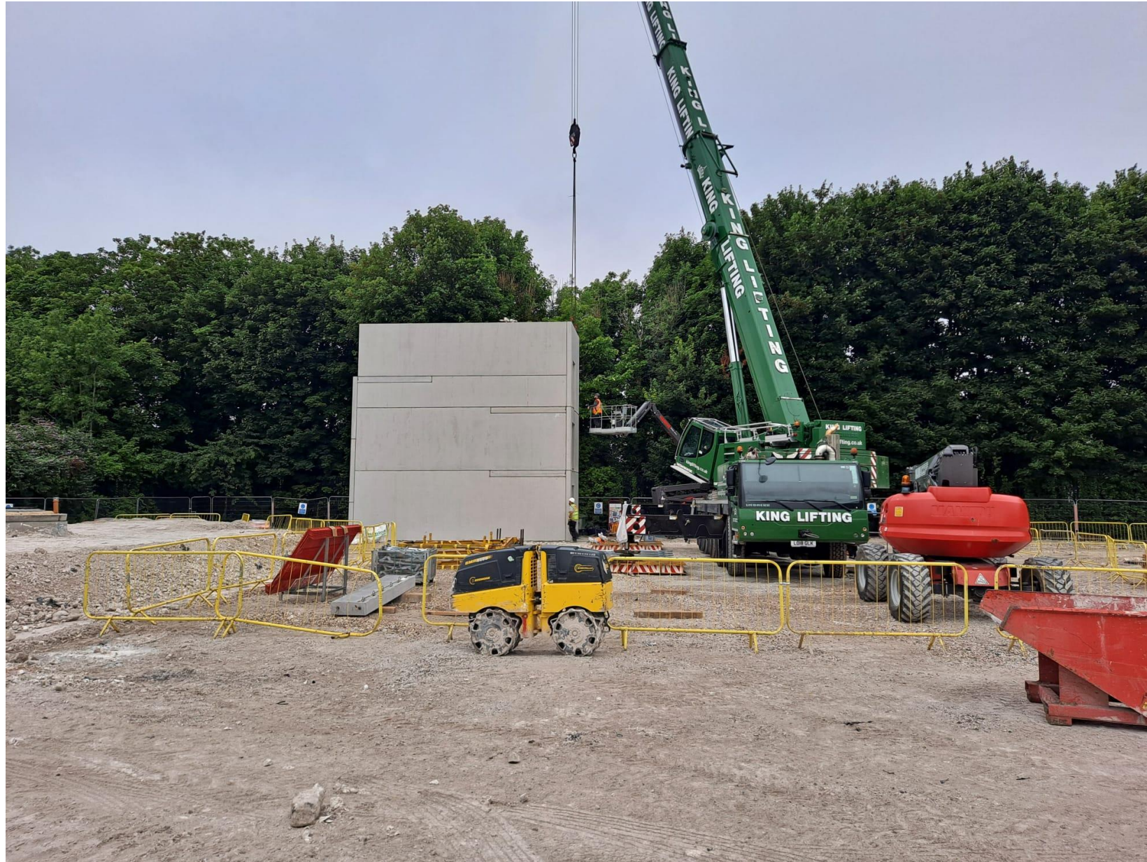
View of stairwell core at full height of 10.225m
